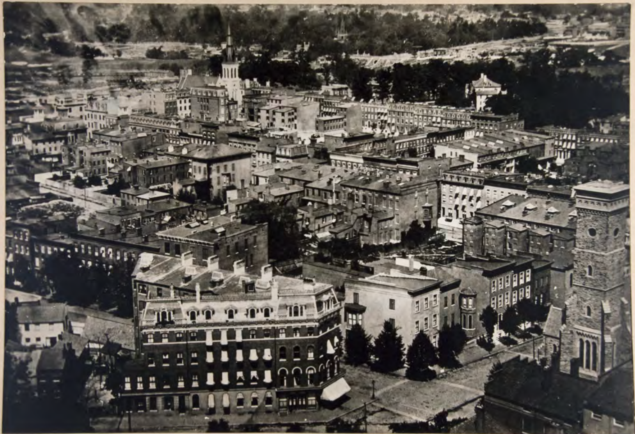
Baltimore, Maryland, circa 1873, looking northwest
